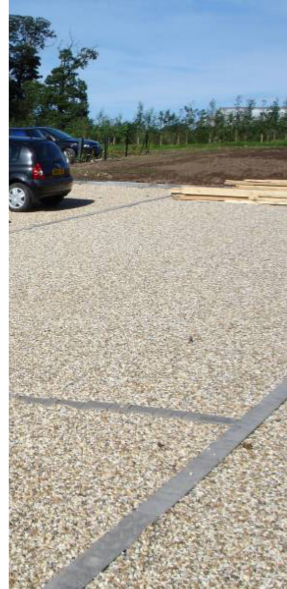
Flush Grade A hardwood timber edge to seperate 'shared zone' from 'pedestrian zone'
