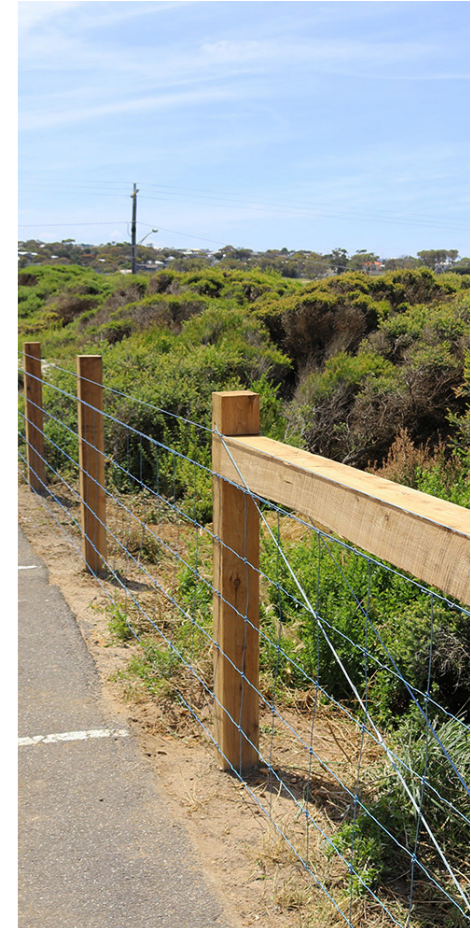
New cypress pine and long life fence to central island planting zone.
