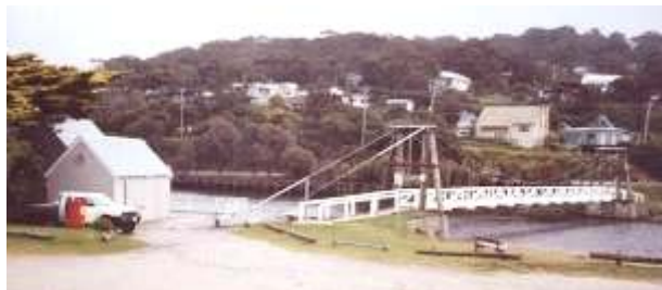
Swing Bridge at Lorne
