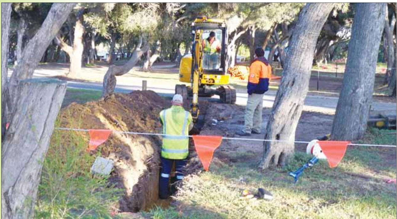
A major power upgrade in the southern half of Torquay Foreshore Caravan Park started in May 2010 with trenches dug (below) and conduit laid (above).
