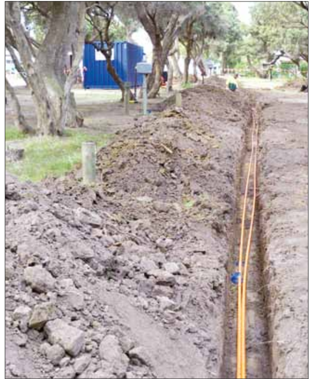
A major power upgrade in the southern half of Torquay Foreshore Caravan Park started in May 2010 with trenches dug (below) and conduit laid (above).
