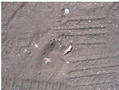
Parking on a midden adjacent to Inlet Crescent. The parking area and paths need to be redefined.
