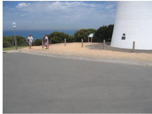
The lighthouse surrounds suggest a space for cars, whereas this is a space for people. The expanse of asphalt also diminishes the lighthouse's beauty.
