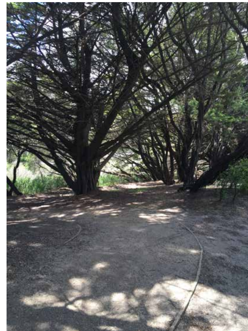
Pedestrian pathways located adjacent to the Erskine River are depleted of gravel toppings and have steep grades making it difficult for pedestrians to safely navigate the pedestrian paths.
