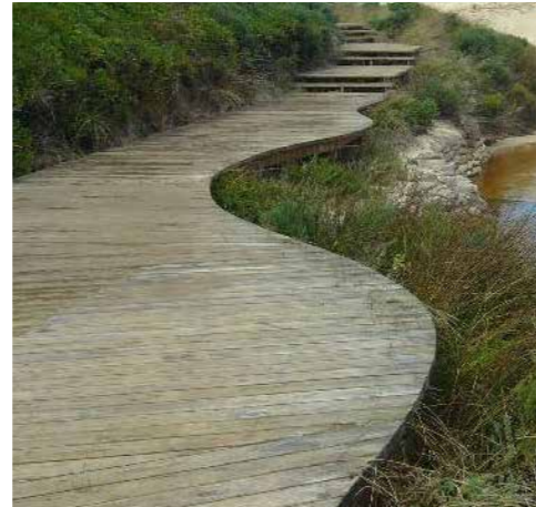
D.2 Timber boardwalk following form of embankment
