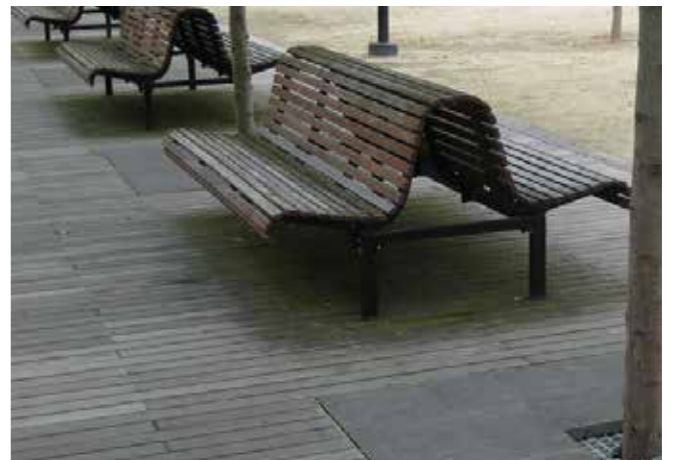
J.9 Timber decking
