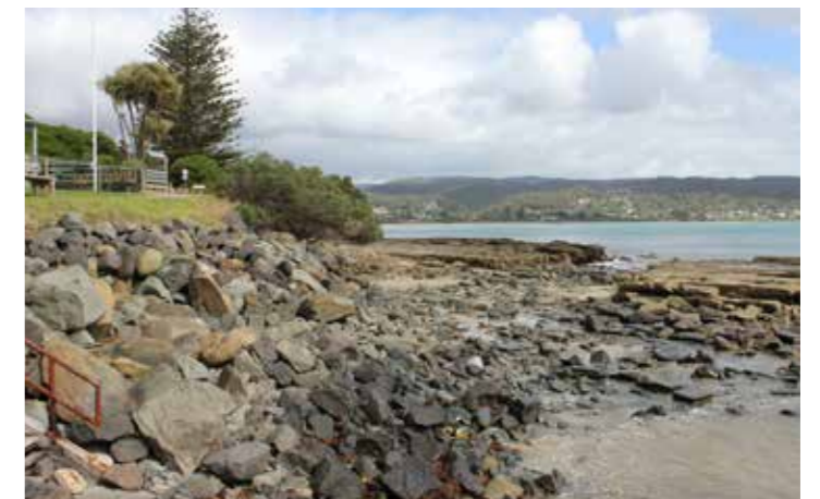
E.4 Existing foreshore edge (rock embankment)
