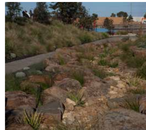
E.3 Rock stabilised embankment, revegetated where possible
