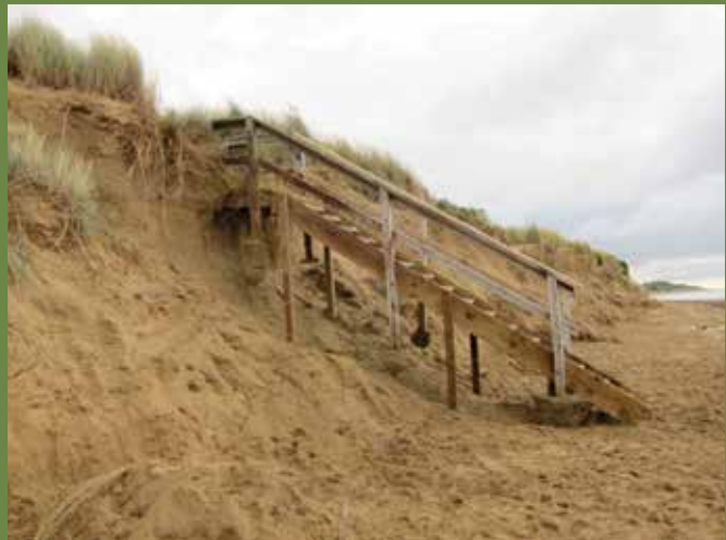
Erosion damage caused to dunes and beach access stairs at White's Beach, Torquay, during storms of May 2011.
