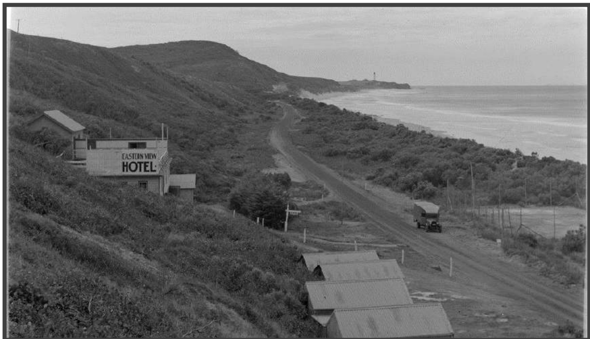
The old Eastern View Hotel, 600 metres east of Coalmine Creek ( Rose Series photograph 1920 to 1954).
