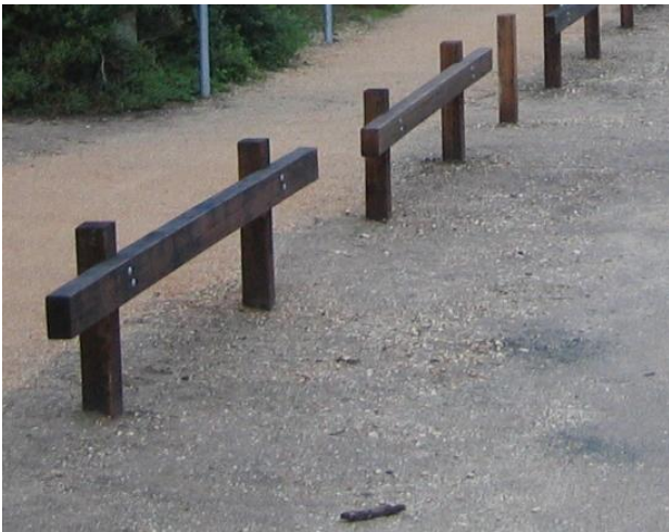
Image 7: Timber post and rail barriers ('H' barriers) prevent vehicle encroachment and help define parking bays without line marking.
