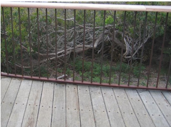
Image 6: Thin, dark coloured railings minimise visual impact, while hardwood timbers suit the tone of the bush.
