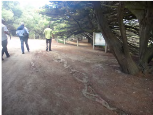
Erosion of gravel paths following periods of heavy rain washing in to the Erskine River.
